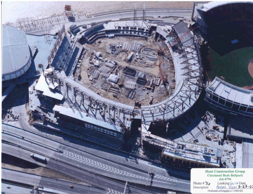
Cinergy Field/Great American Ball Park Construction - 2002
