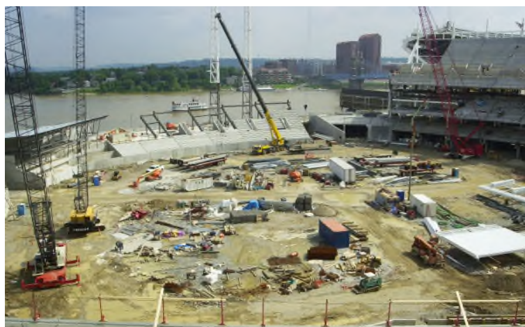
Figure 13 Great American Ball Park Superstructure Construction
