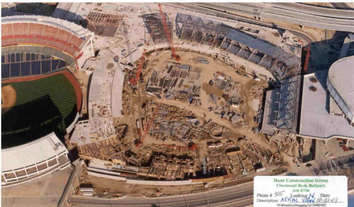
Cinergy Field/Great American Ball Park Construction - 2001
