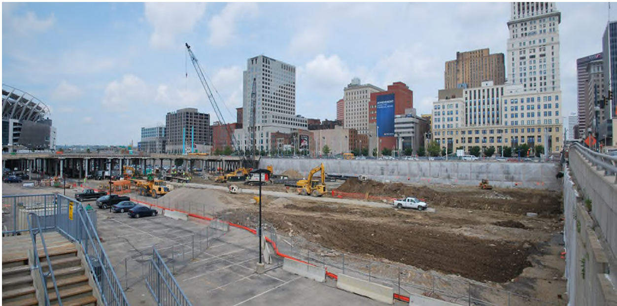
Figure 2- Phase II Public Infrastructure Construction: 2010
