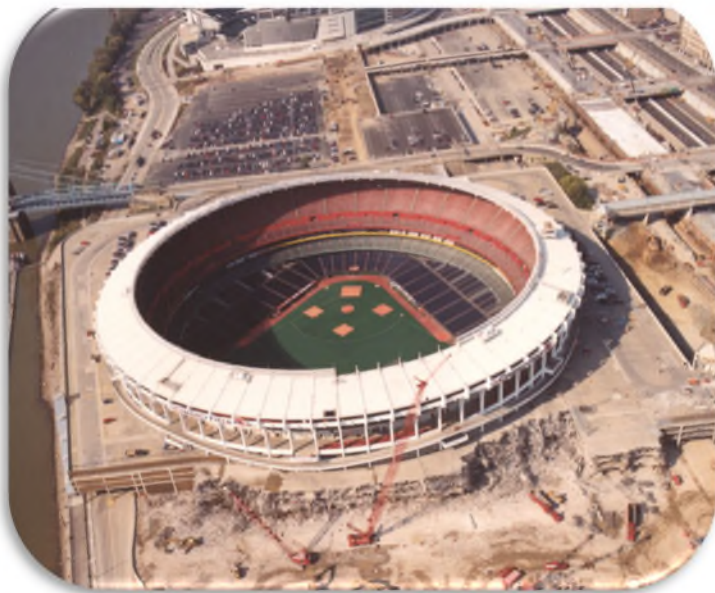
Cinergy Field Partial Demolition: 2001
