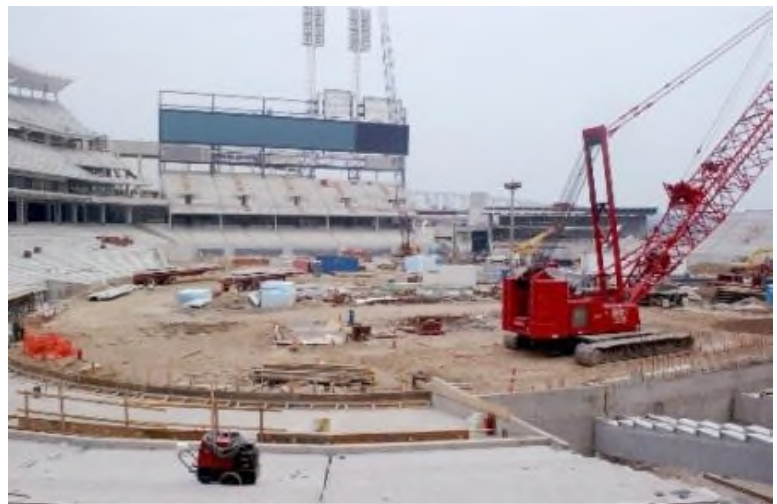
Great American Ball Park Superstructure Construction
