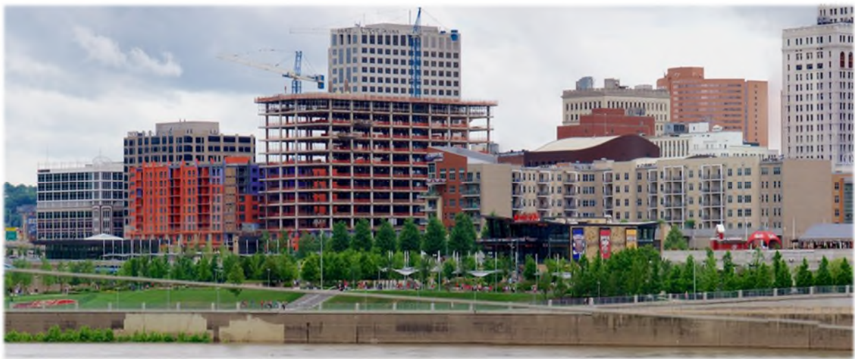
Figure 8 GE Global Operations Center and Podium Under Construction: 2015-2016
